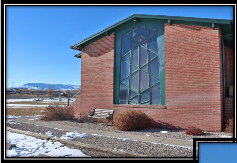
East Side of Building Facing Parking Area
